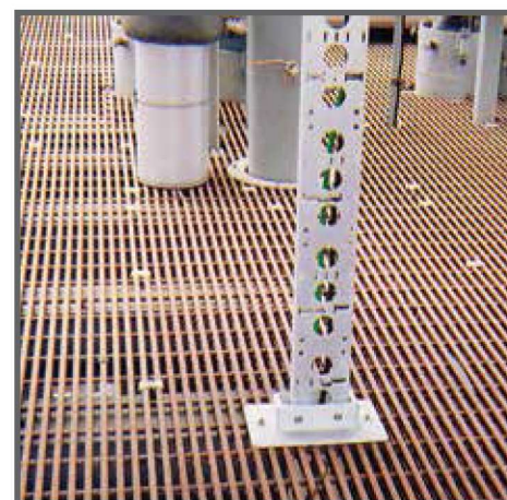
Offshore Oil & Gas Platform
